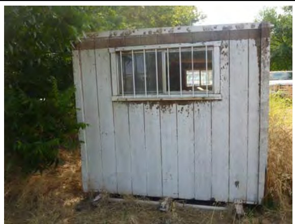
Photo 12: A structure without a foundation within the project area was observed.
